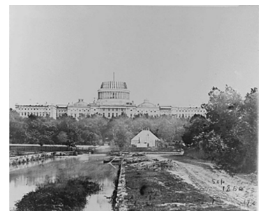
The U.S. Capitol under construction, 1860 (National Archives Identifier 530494) www.loc.gov
